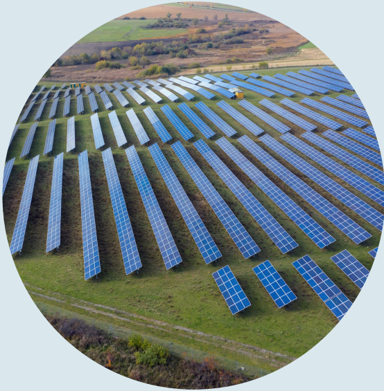
Hilly Solar Farm
